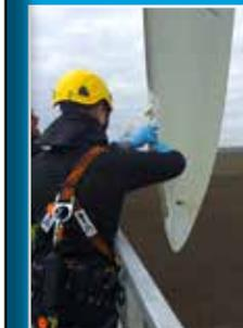
The quick and easy set up of the truck mount, along with the skill of the operator, allowed the technicians to inspect and repair all three blades on the turbine in one day, minimising the lost production for the turbine owner.
